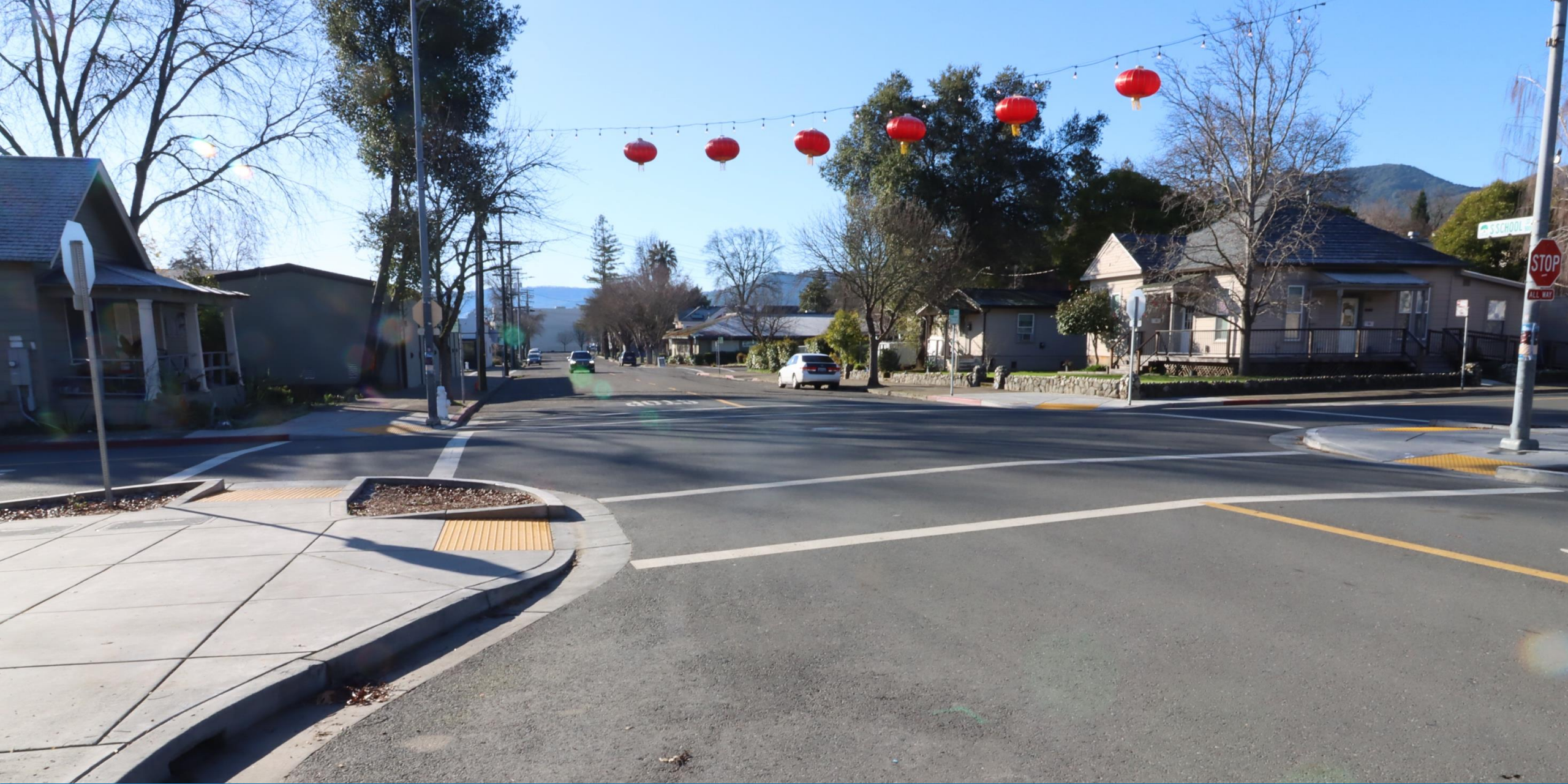
Newer sections of School Street have 2 ramps per corner and curb extensions. Many 4-way stops help keep speeds low.
