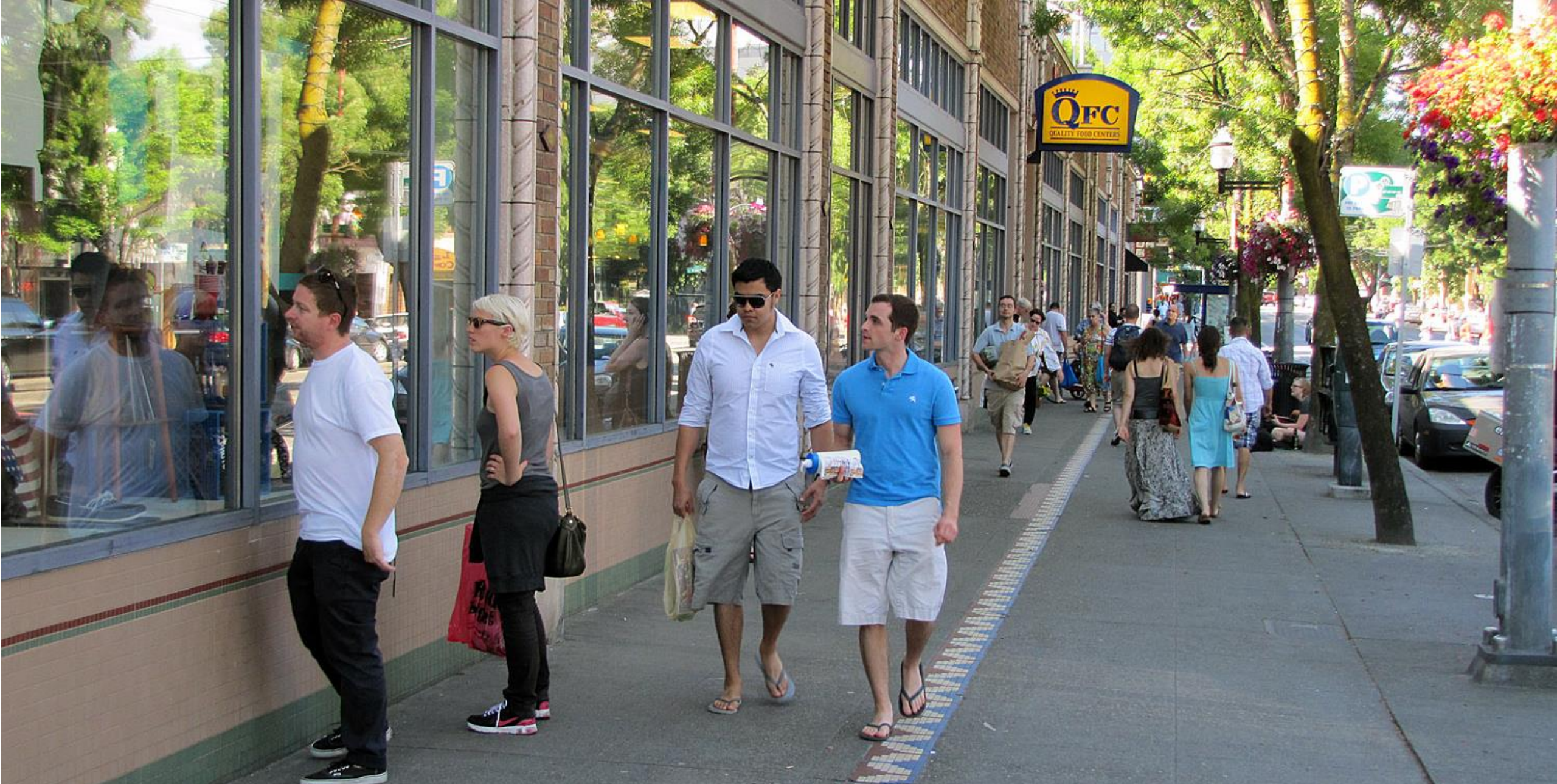
To fully activate a street ground floor window glazing should fall within the range of 70-90%
