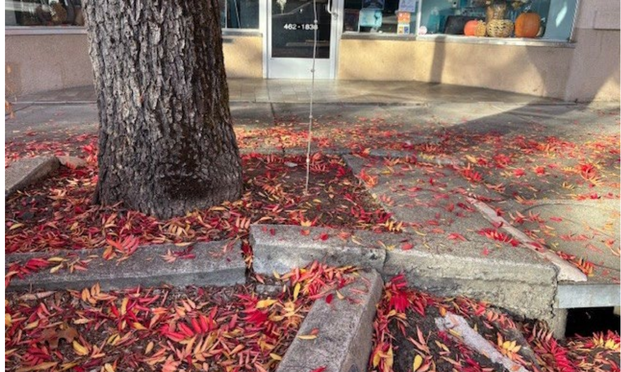
Improperly planted trees cause multiple problems, from drainage, to uplifting curbs, to cracked building foundations.
