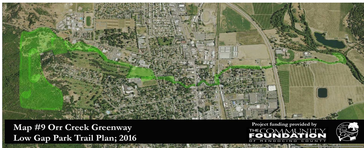
Figure. 2 Orr Creek Greenway
