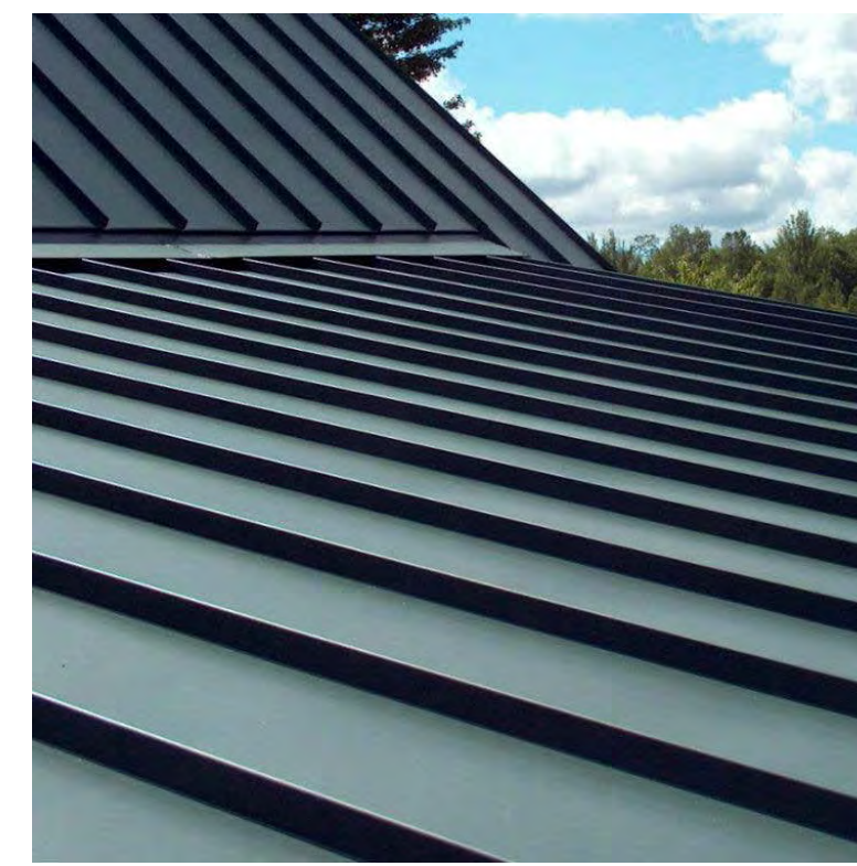
VERTICAL SEAM METAL ROOF METAL SALES - CLASSIC GREEN
