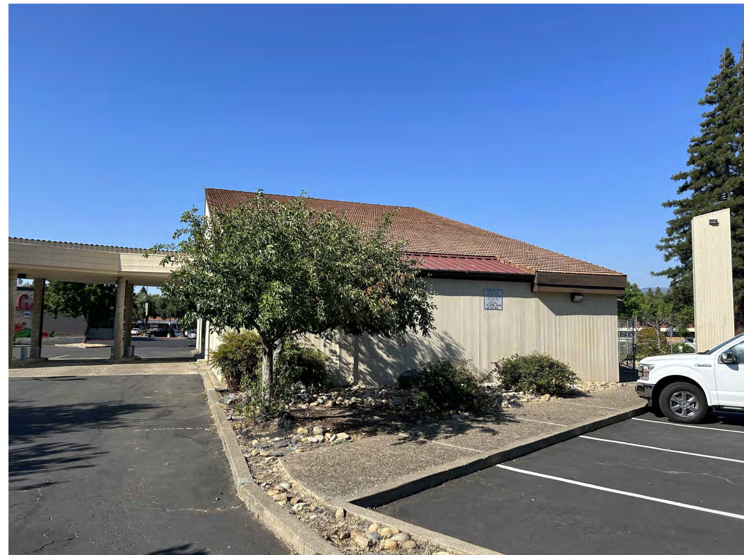
(FRONT WALL; SOUTH SIDE)
