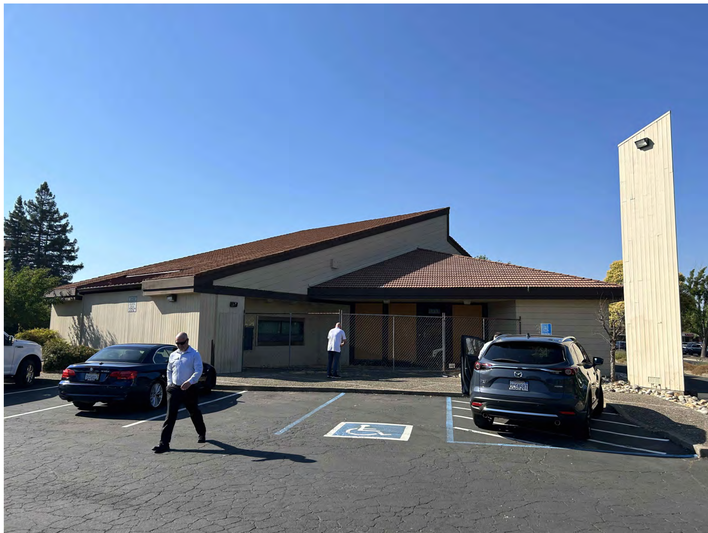
(FRONT ENTRY; SOUTH SIDE)
