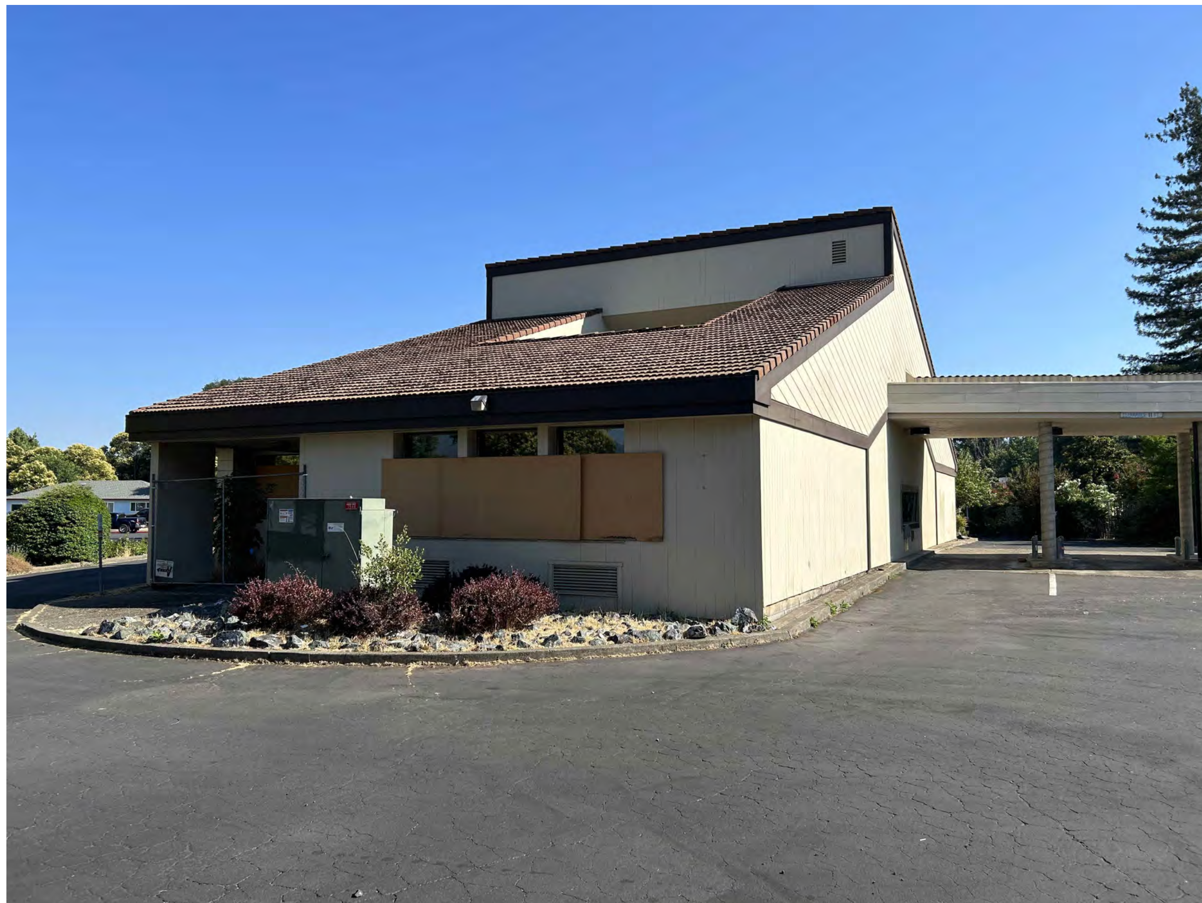
(BACK WALL; NORTH SIDE)
