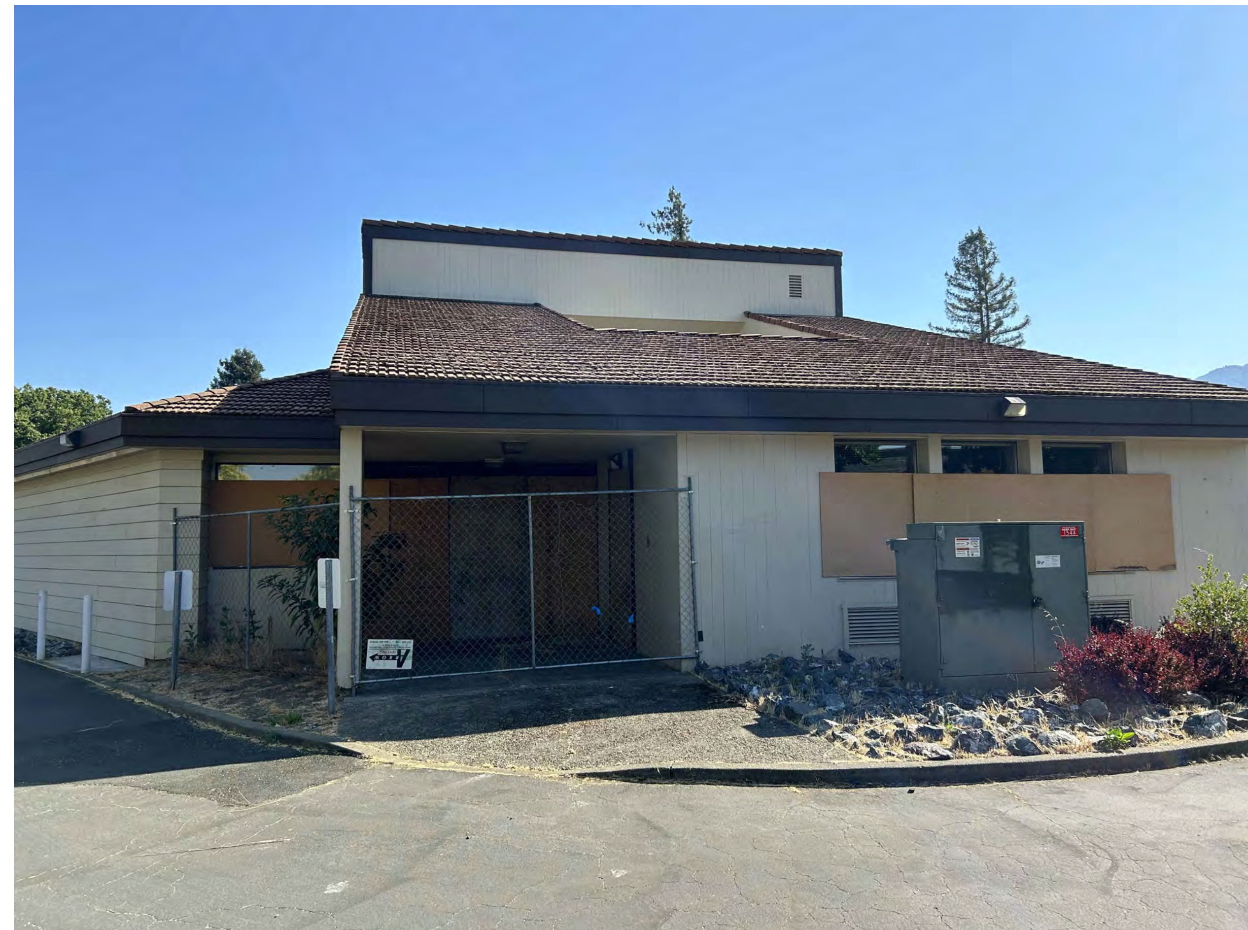
(BACK ENTRY; NORTH SIDE)
