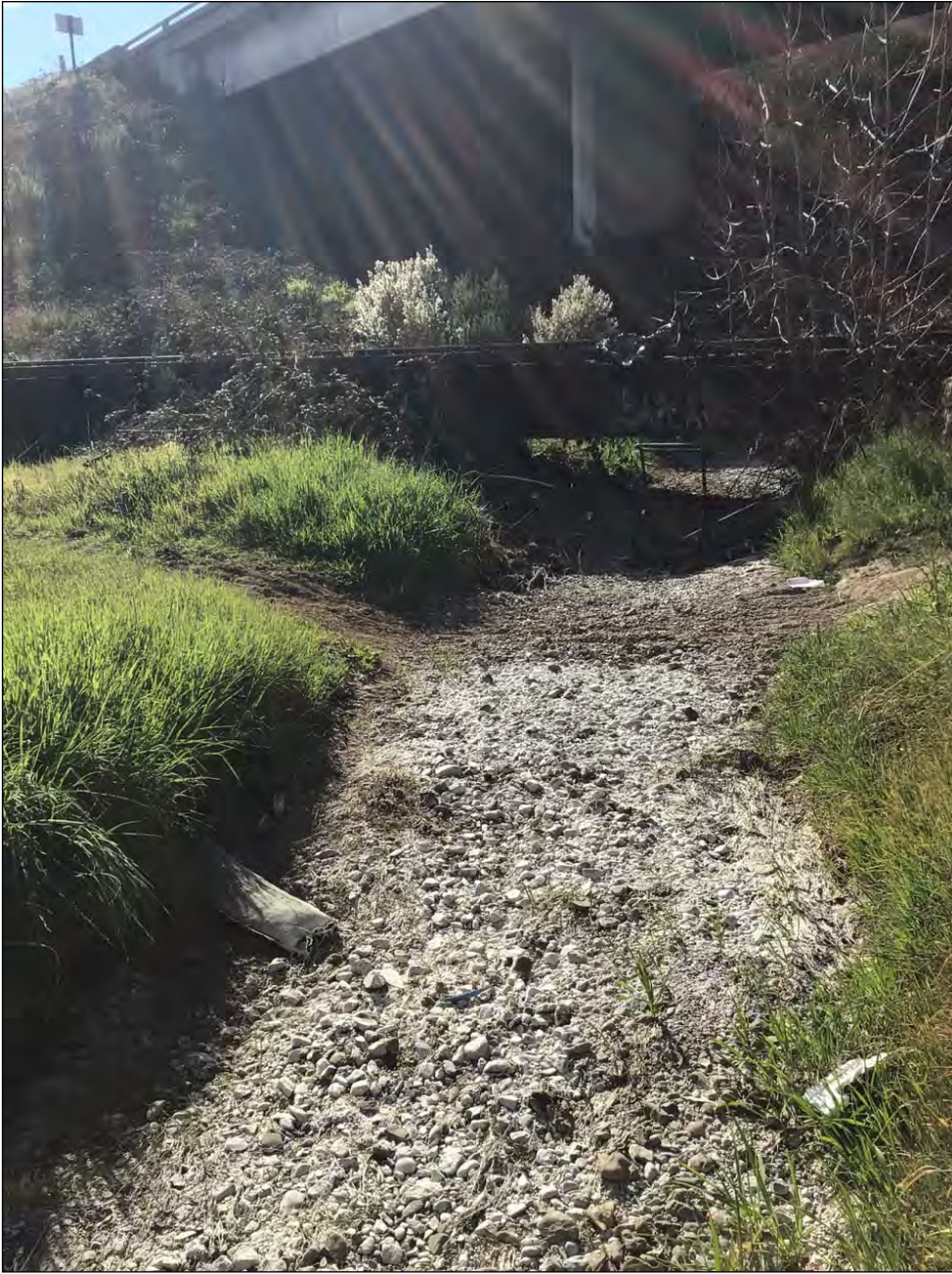
Photo 5: Drainage D-2 near Highway 101. Photo looking west.
