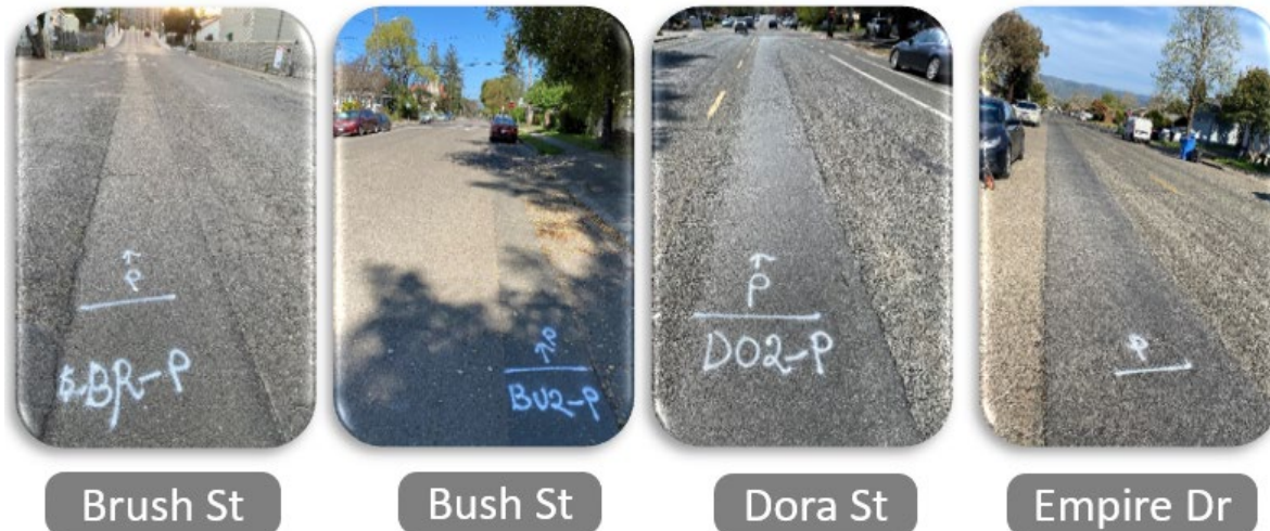
Figure 19. Typical Full-Block Trench Cuts in Ukiah
