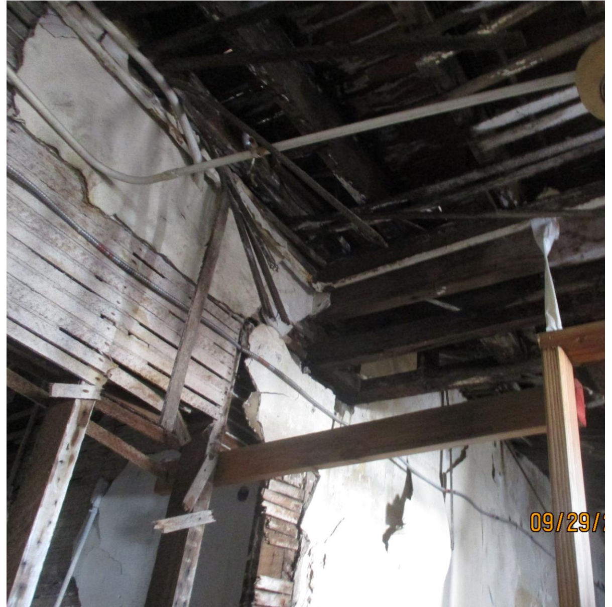
2 ND FLOOR FIRE HAZARD EXPOSED WOOD
