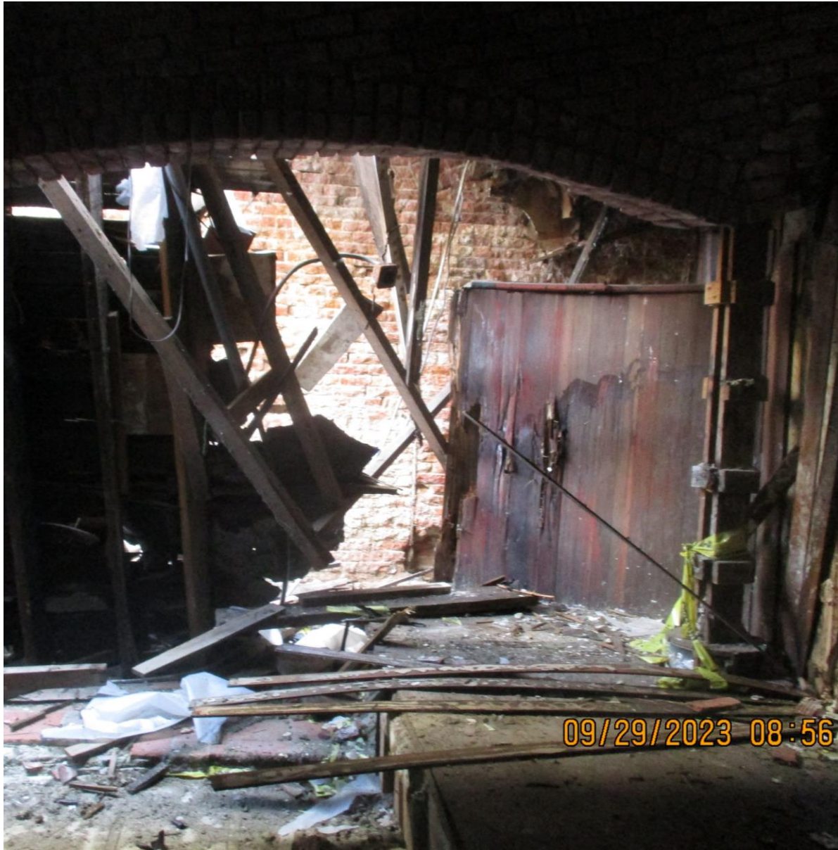
1 ST FLOOR: 2 ND FLOOR STRUCTURAL FAILURE
