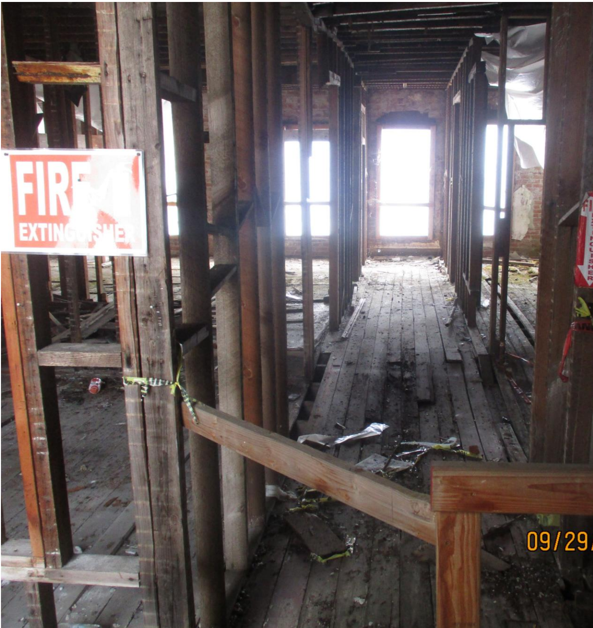
3 RD FLOOR UNEVEN AND COMPROMISED, STATE. DRY-ROT FLOOR ALSO COMPROMISED, STRUCTURAL FAILURE
