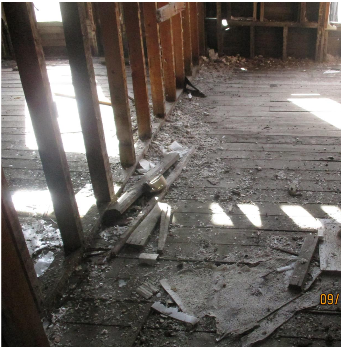
3 RD FLOOR UNEVEN AND COMPROMISED, SMITH/STATE . DRY-ROT FLOOR ALSO COMPROMISED, STRUCTURAL FAILURE
