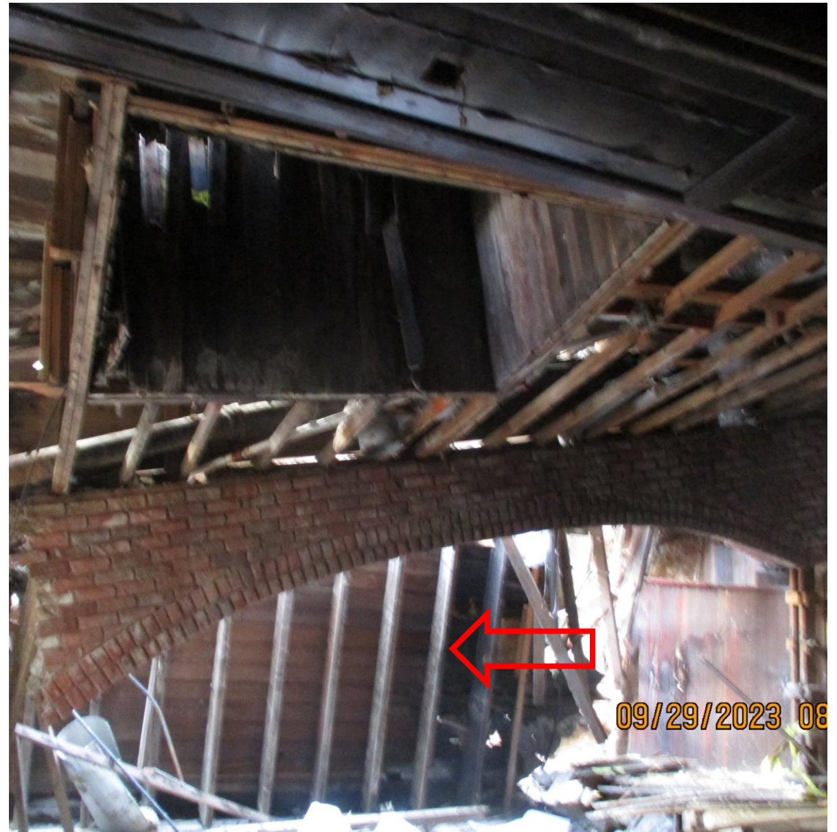
ROOF FROM ABOVE 2 ND FLOOR
