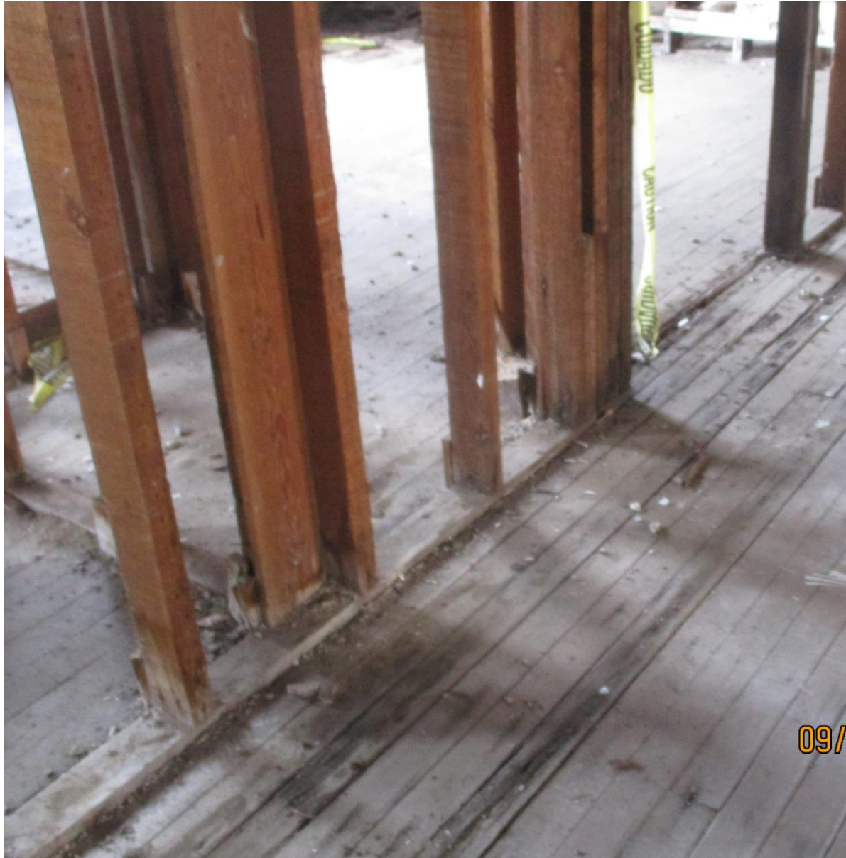
2 ND FLOOR UNEVEN AND COMPROMISED, SMITH ST SIDE. DRY-ROT FLOOR ALSO COMPROMISED
