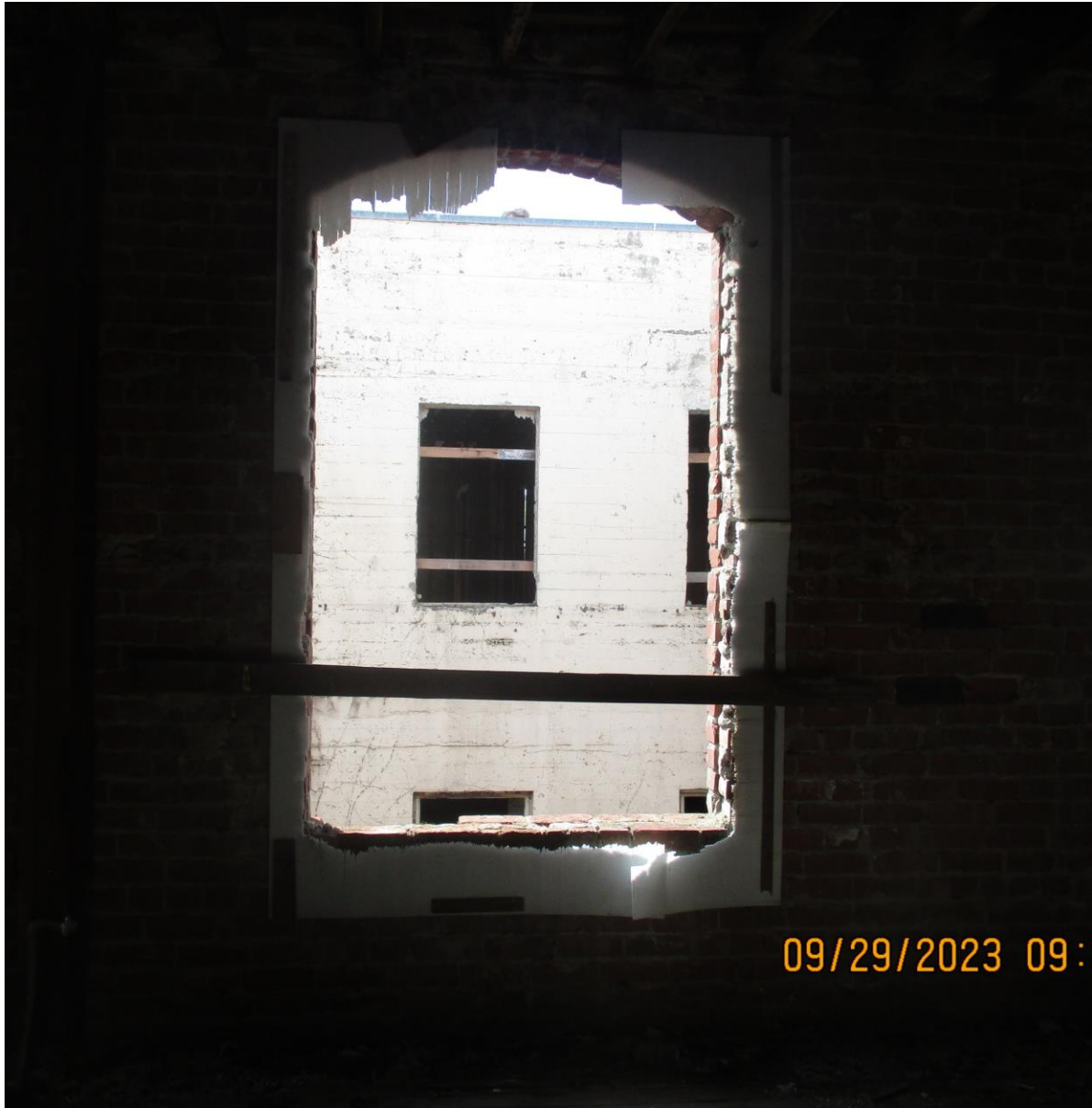
3 RD FLOOR: OPEN TO WEATHER
