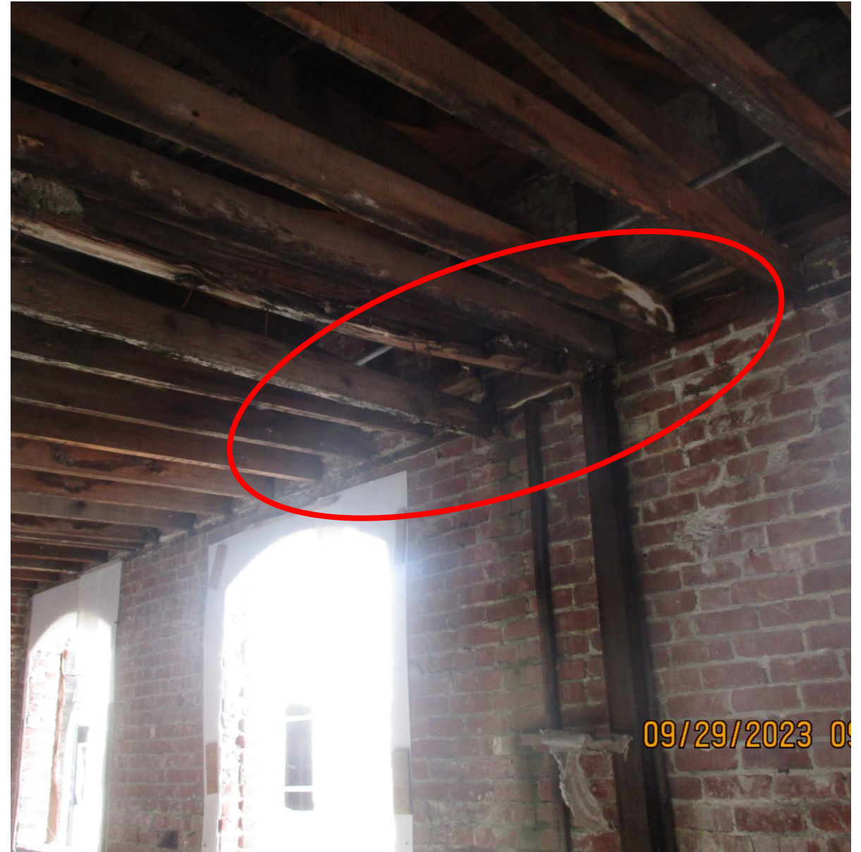
3 RD FLOOR UNEVEN AND COMPROMISED, SMITH ST SIDE. DRY-ROT FLOOR ALSO COMPROMISED, STRUCTURAL FAILURE
