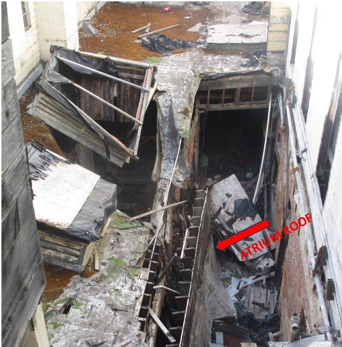
3RD FLOOR COLLAPSED ATRIUM FROM ABOVE
