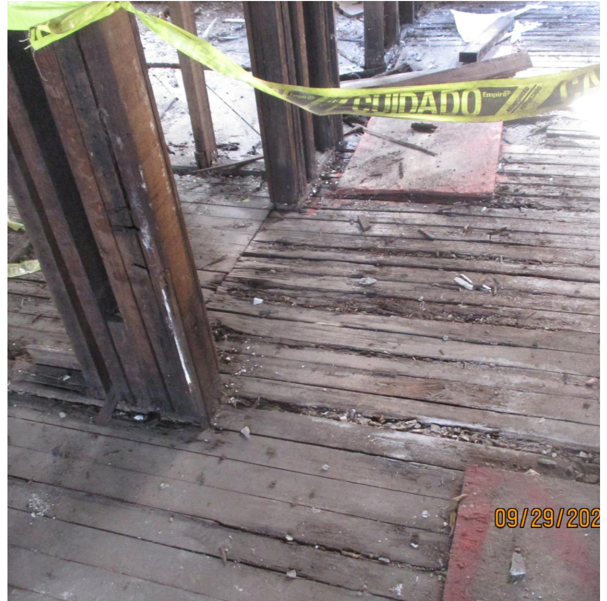
2 ND FLOOR UNEVEN AND COMPROMISED, SMITH ST SIDE. DRY-ROT FLOOR ALSO COMPROMISED
