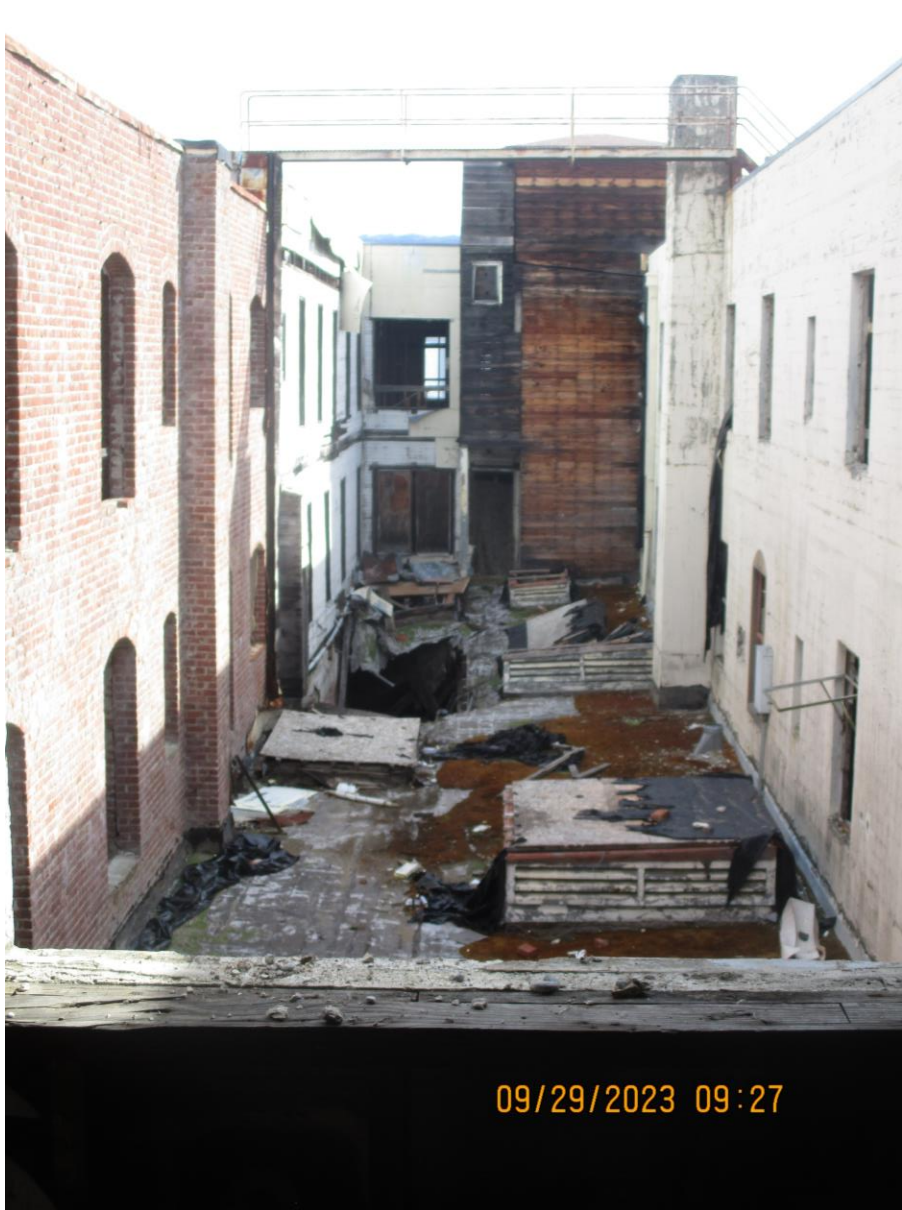
3 rd FLOOR LOOKING AT 2 ND FLOOR ATRIUM. FLOOR JOIST/ROOF STRUCTURAL FAILURE
