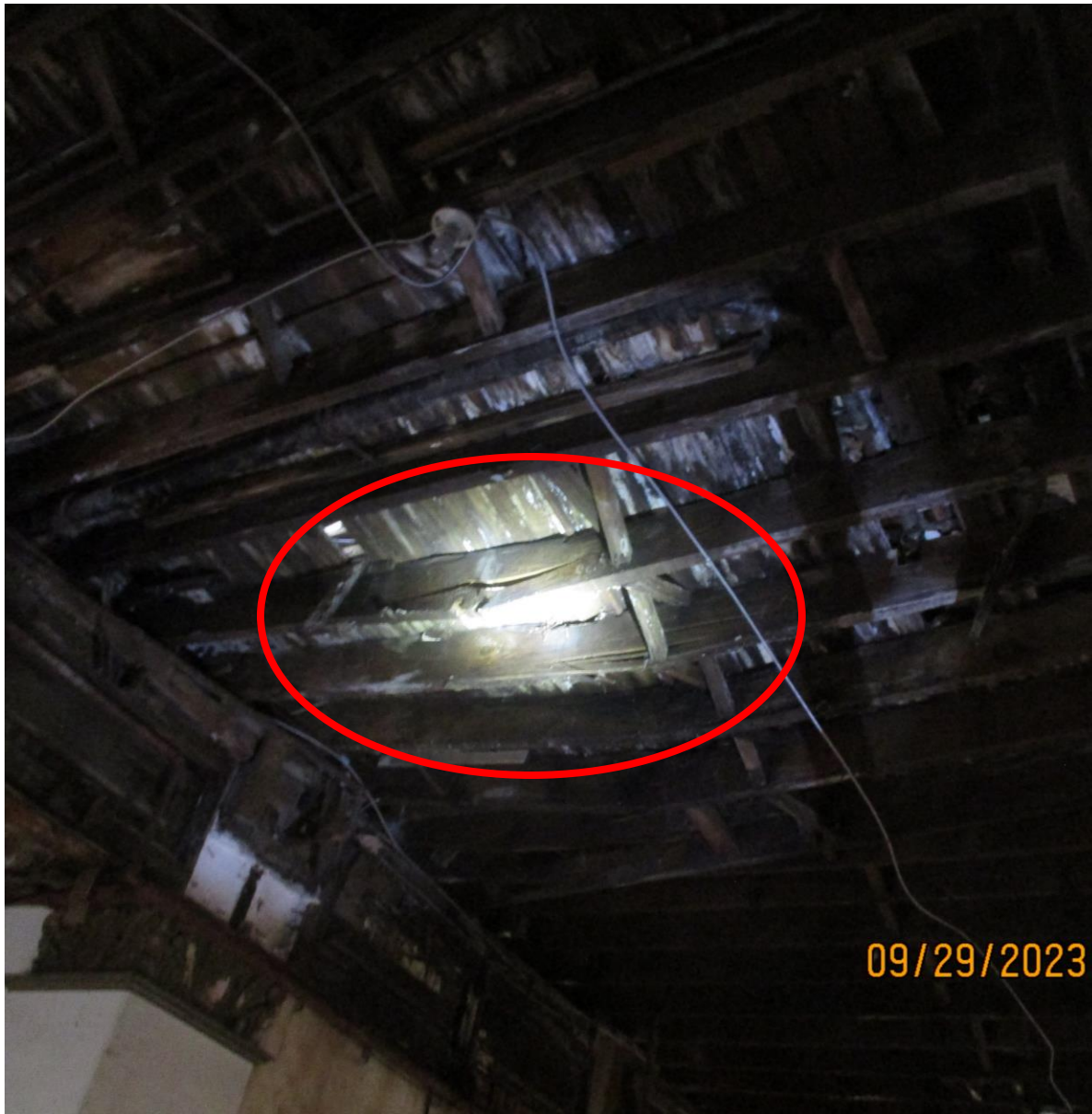
1 ST FLOOR LOOKING AT 2 ND FLOOR, AT STATE ST SIDE OF BUILDING. FLOOR JOIST STRUCTURAL FAILURE
