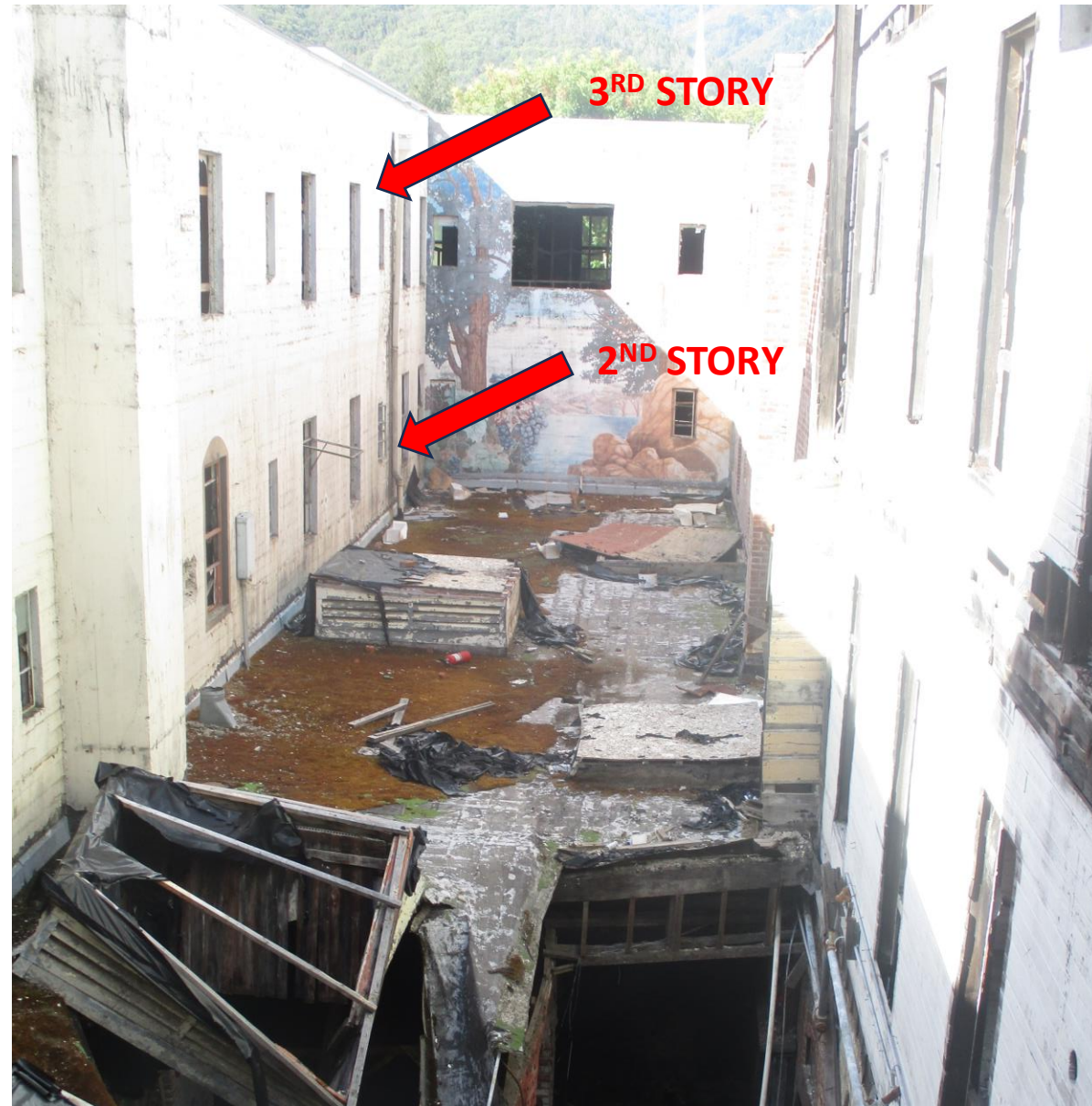
3RD FLOOR COLLAPSED ATRIUM FROM ABOVE
