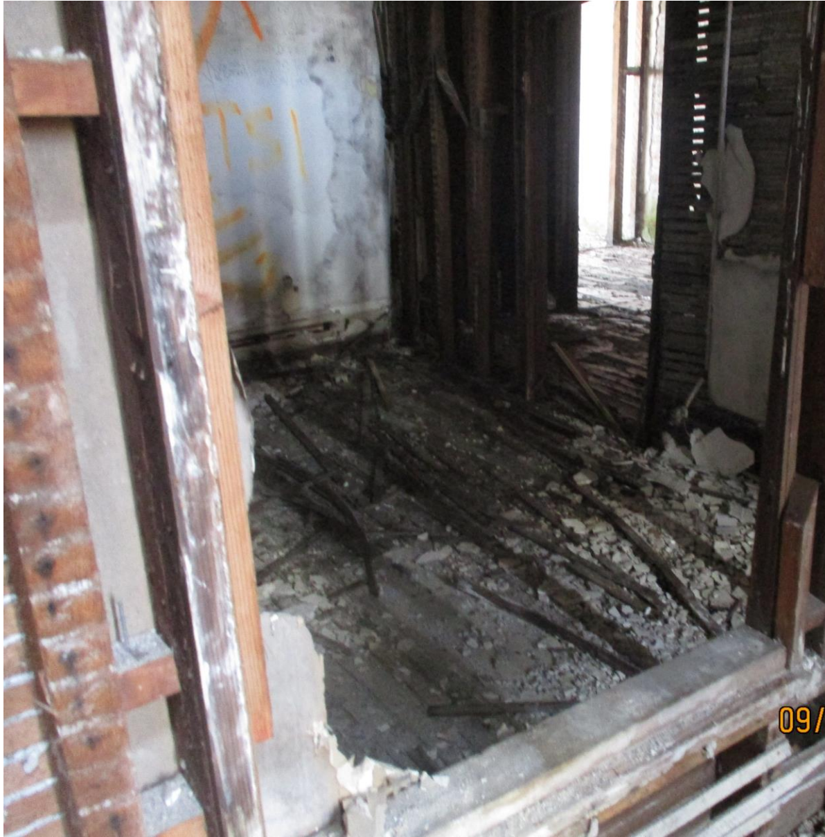
2 ND FLOOR FIRE HAZARD EXPOSED WOOD
