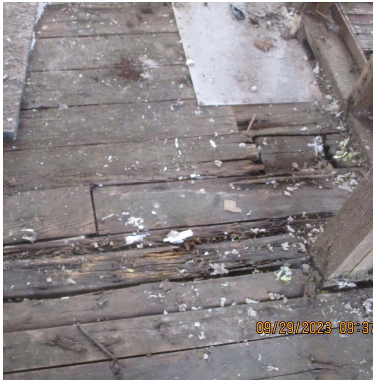
3 RD FLOOR UNEVEN AND COMPROMISED, SMITH/STATE . DRY-ROT FLOOR ALSO COMPROMISED, STRUCTURAL FAILURE
