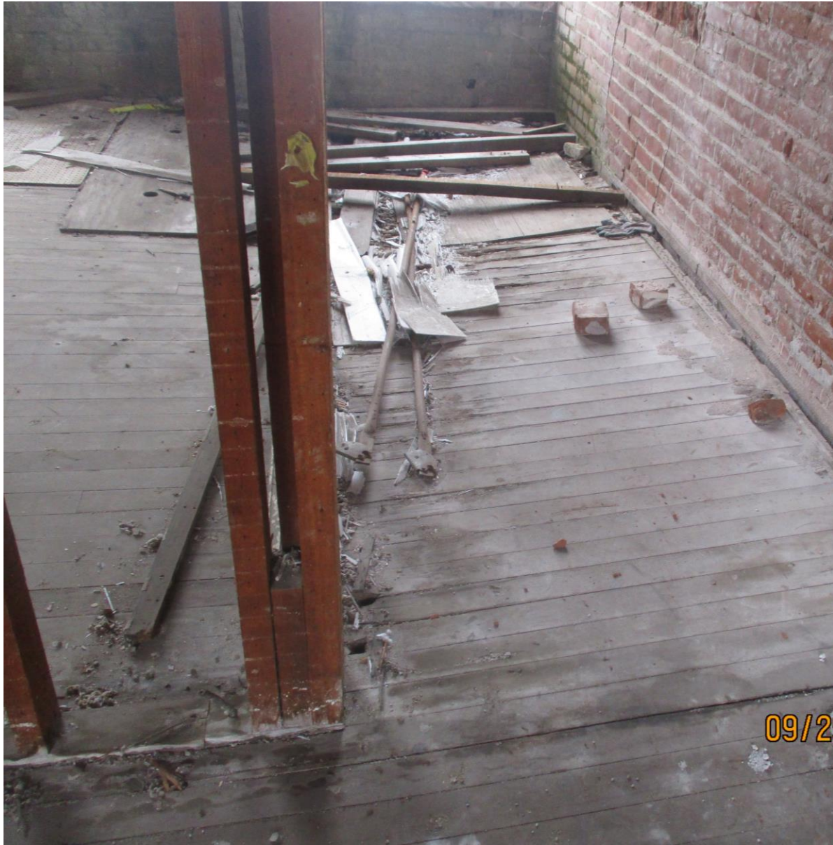
3 RD FLOOR UNEVEN AND COMPROMISED, SMITH ST SIDE. DRY-ROT FLOOR ALSO COMPROMISED, STRUCTURAL FAILURE
