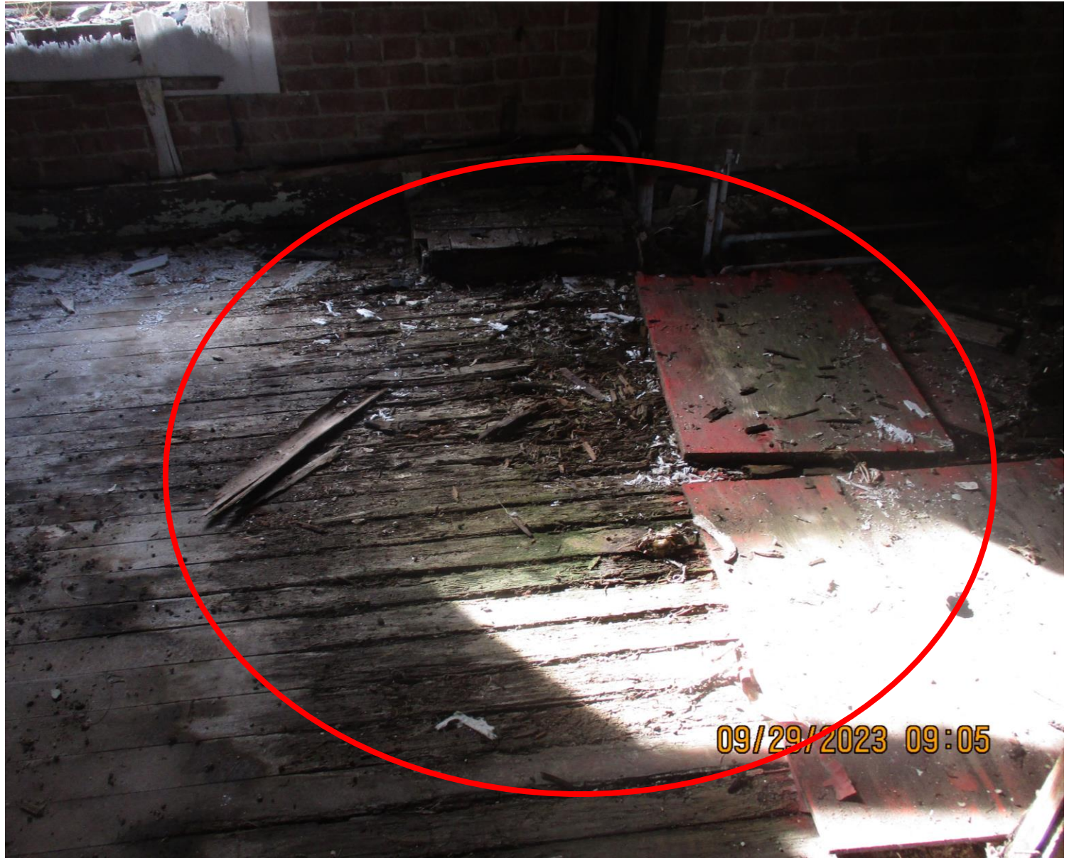
2 ND FLOOR UNEVEN AND COMPROMISED, SMITH ST SIDE. DRY-ROT FLOOR ALSO COMPROMISED
