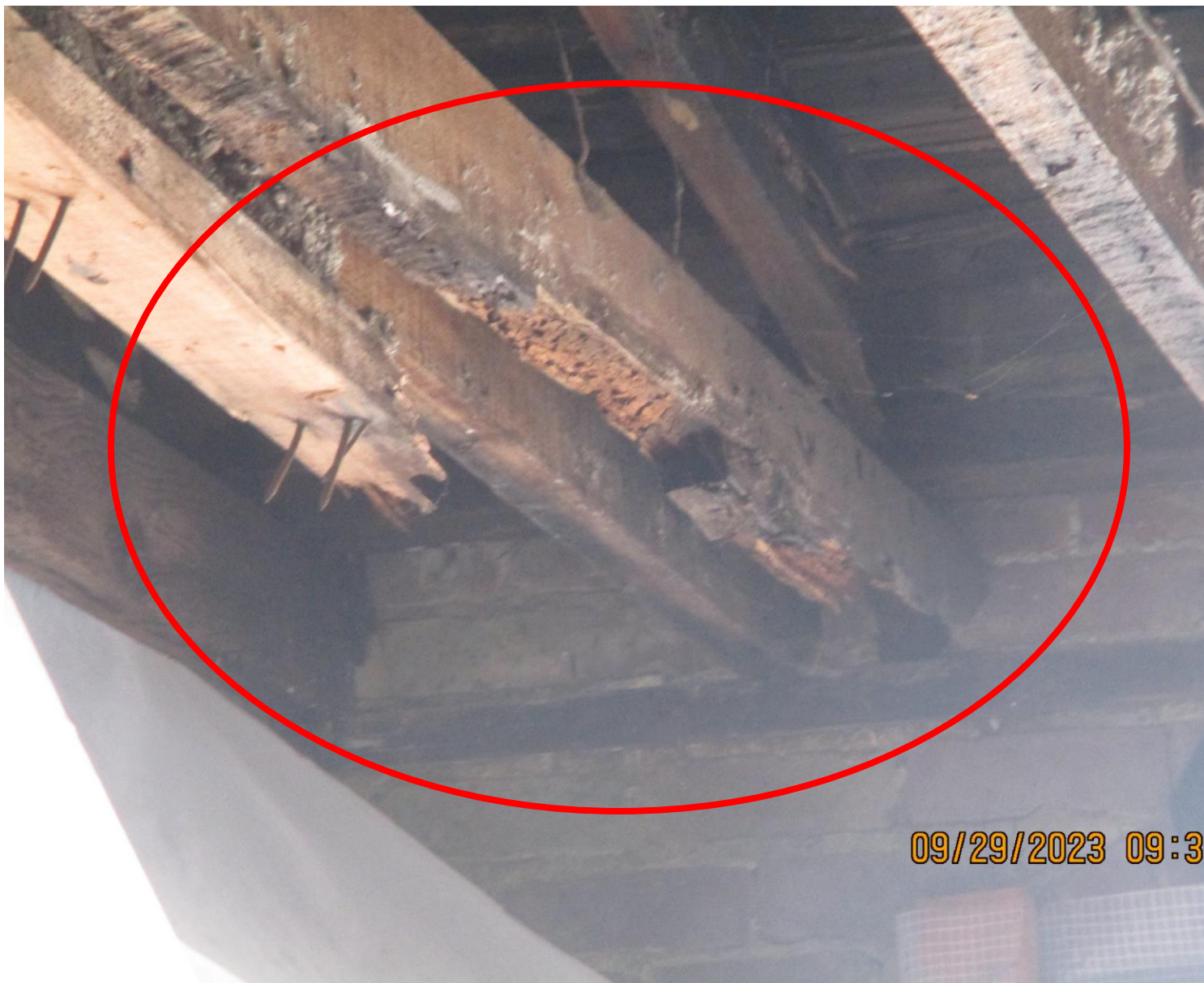
3 RD FLOOR UNEVEN AND COMPROMISED, SMITH ST SIDE. DRY-ROT FLOOR ALSO COMPROMISED, STRUCTURAL FAILURE
