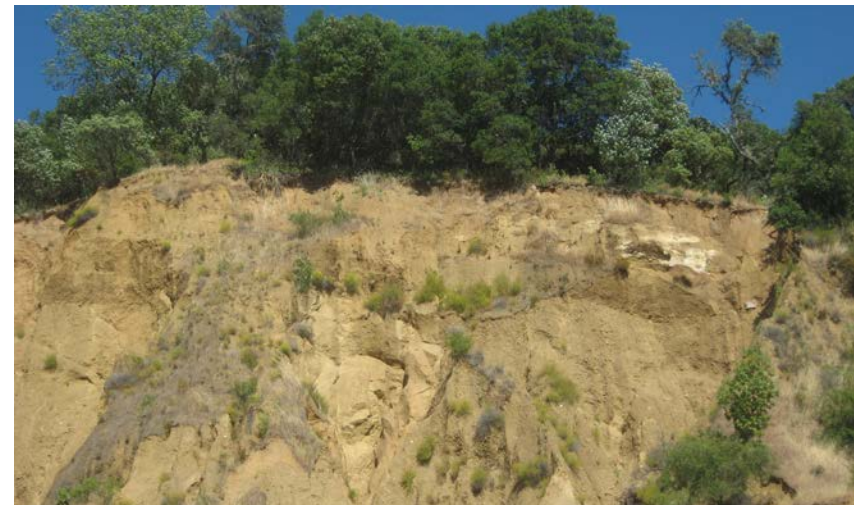
Areas at high risk of erosion along Redemeyer Road.
