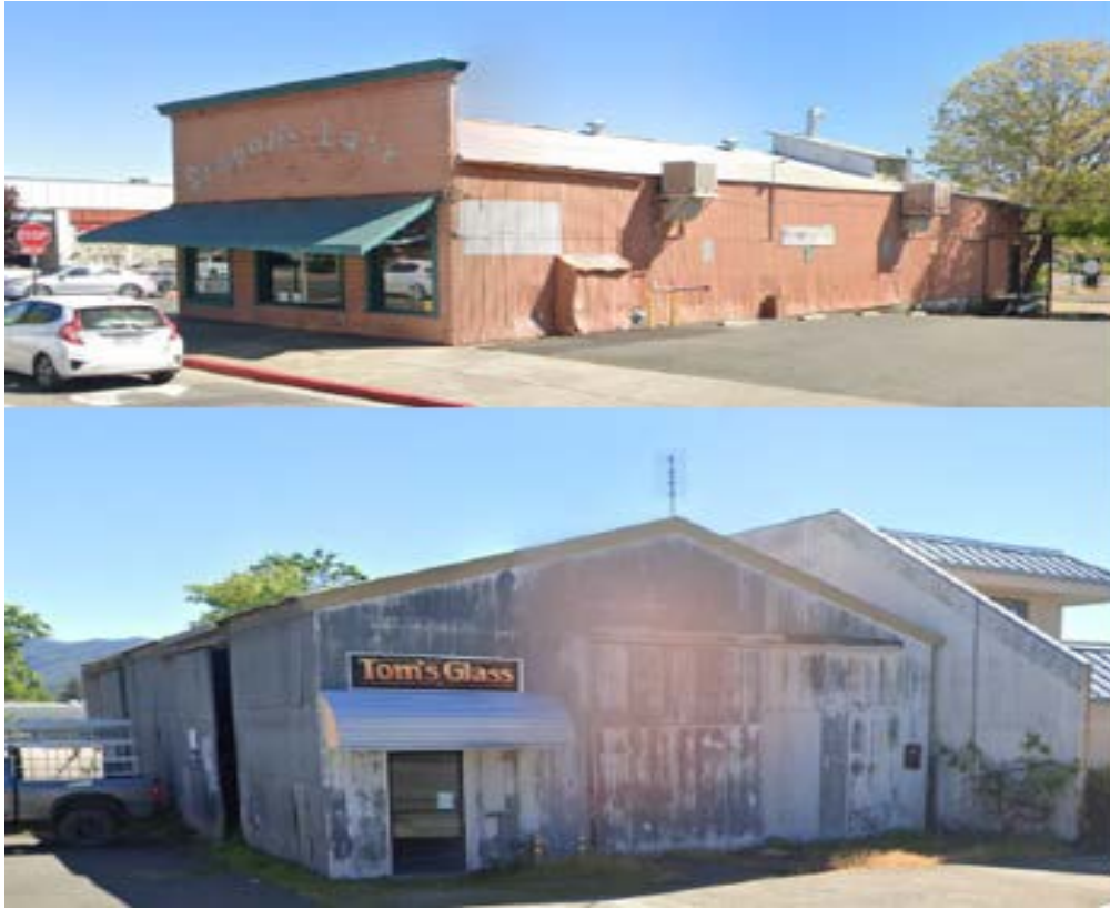
Figure 4, Views of Existing Buildings from S. Main St. (looking northeast)
